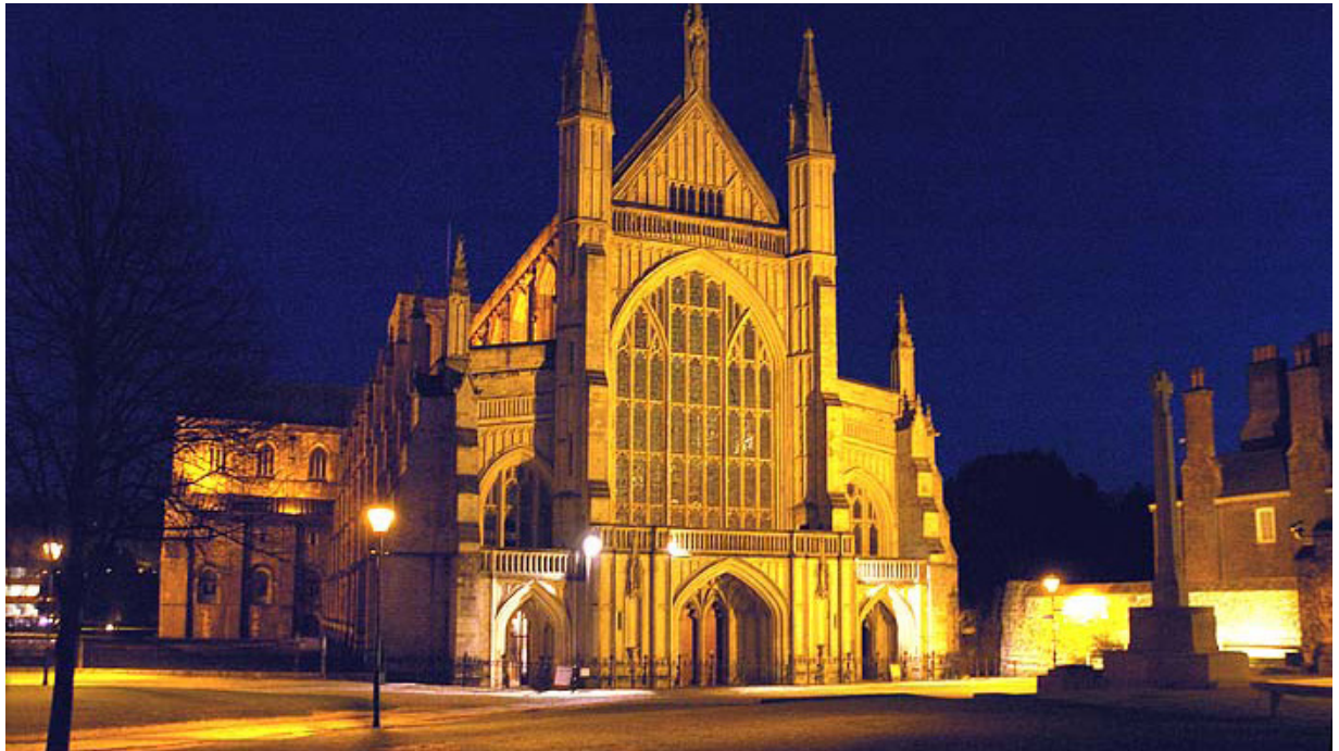
Winchester Cathedral – Specialist Site Wide Lighting Installation & Building Services Upgrade
